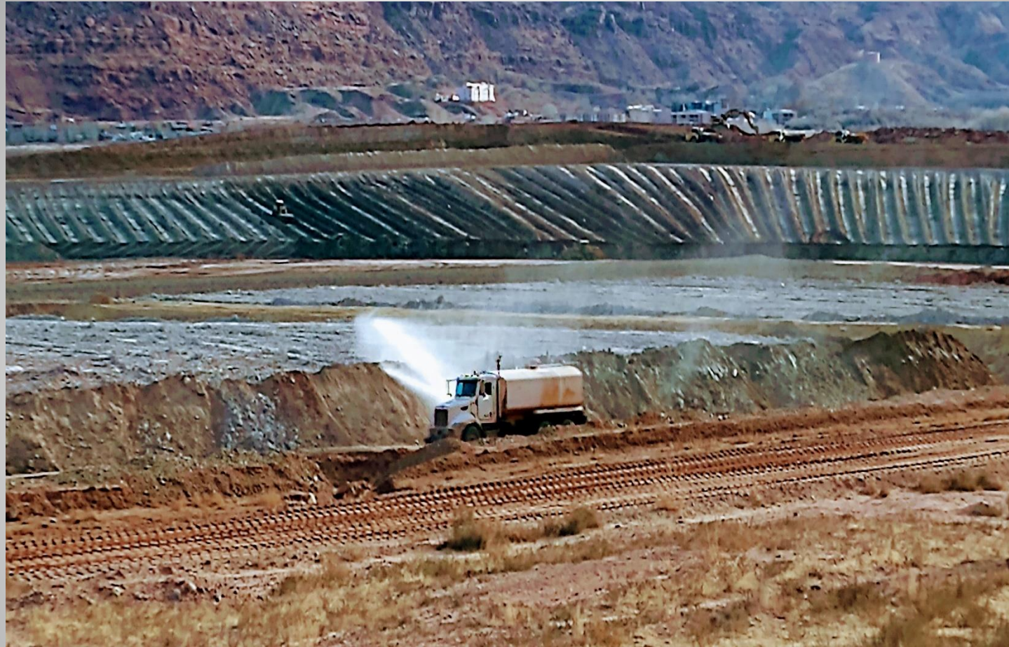
Watering edge of conditioning bed for dust control
