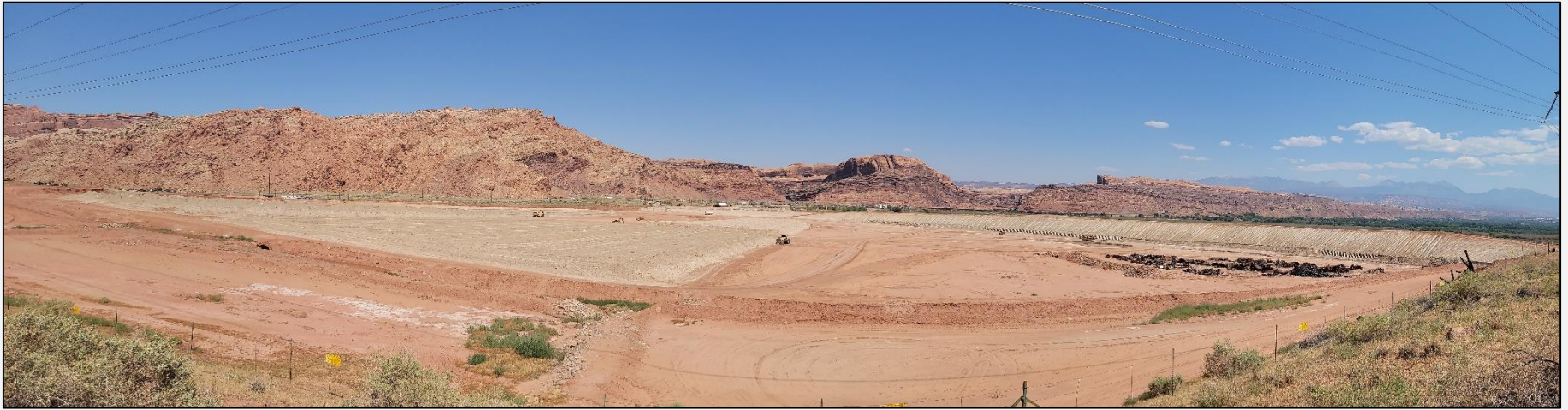
Panoramic view of Moab UMTRA Site (8/29/2022)
