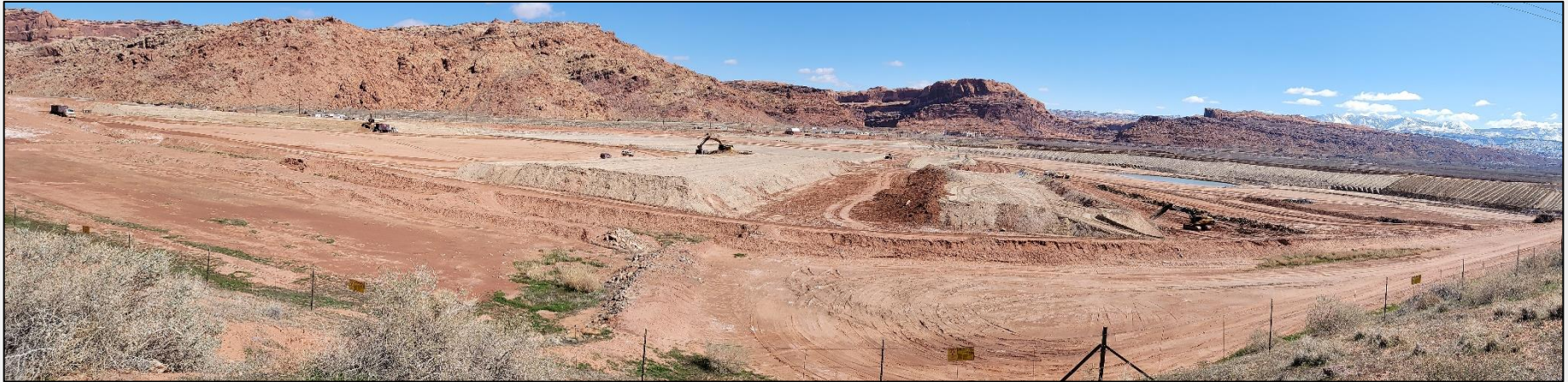
Panoramic view of Moab UMTRA Site (3/27/2023)
