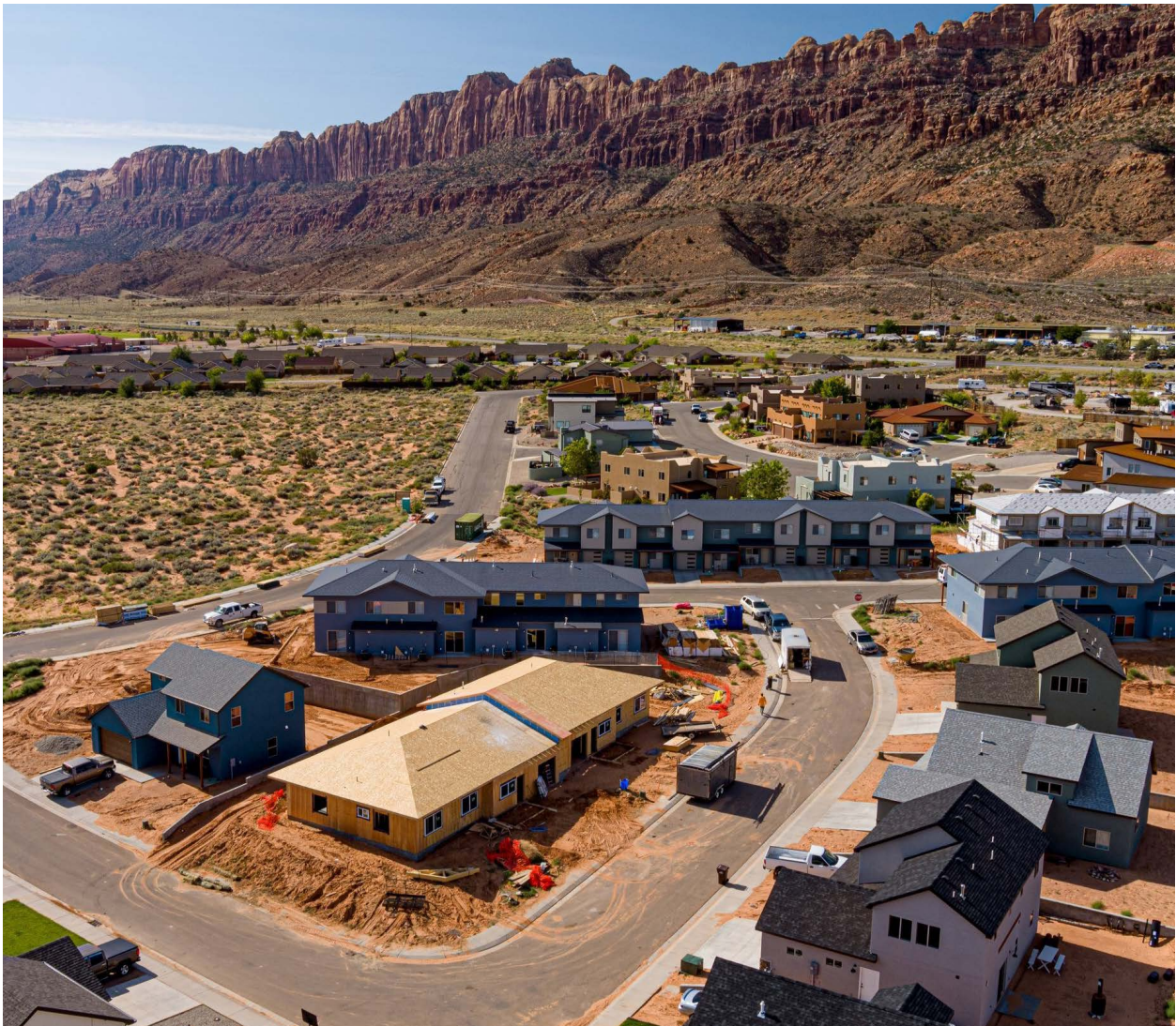
Construction of Wingate Village townhomes in Spanish Valley, 2020.
