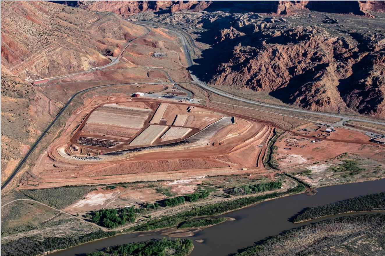
Excavation & conditioning areas
