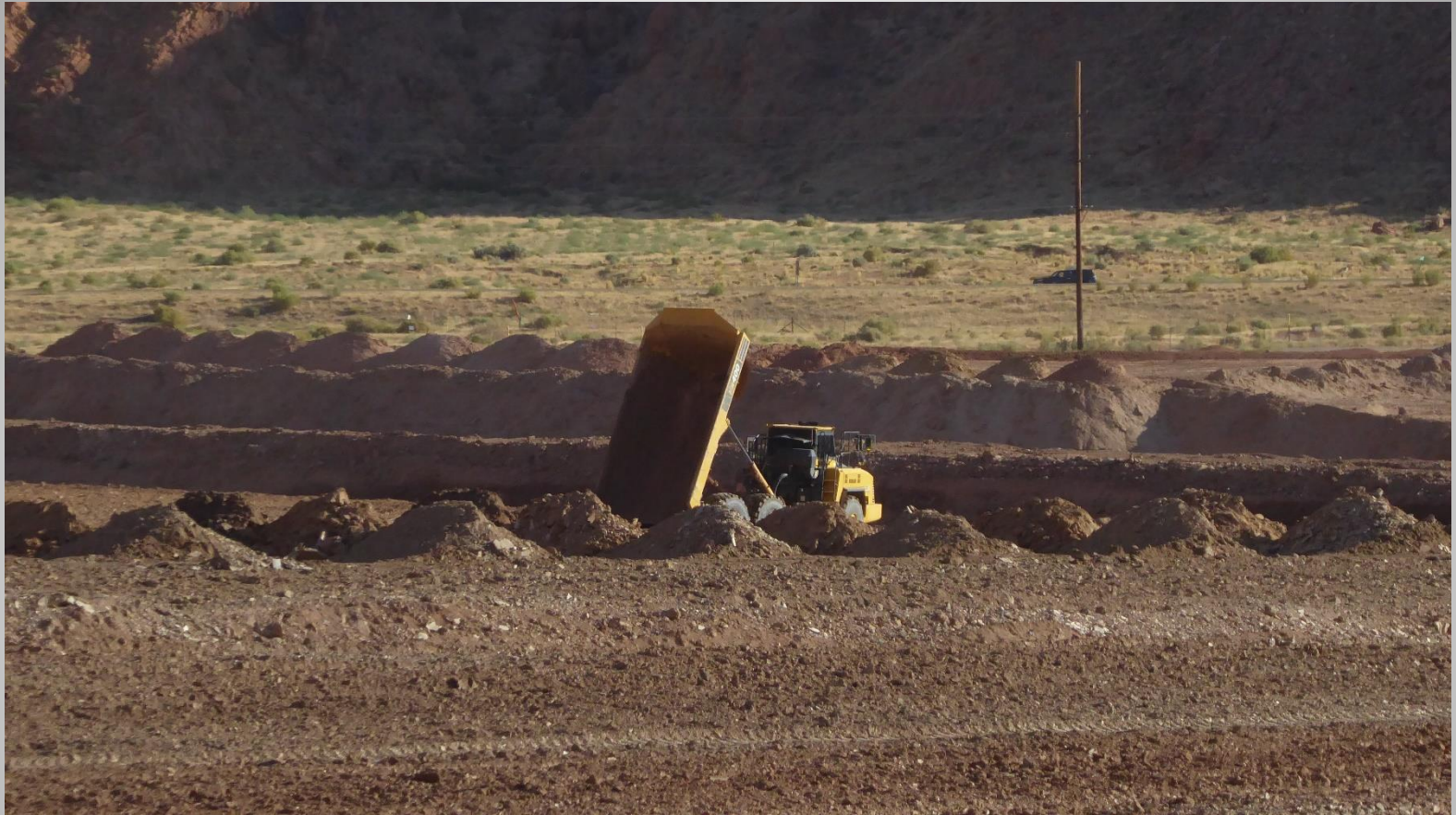
Dumping RRM at one of the multiple conditioning areas
