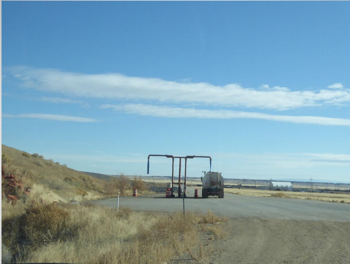
CJ Water loading area below water reservoir.
