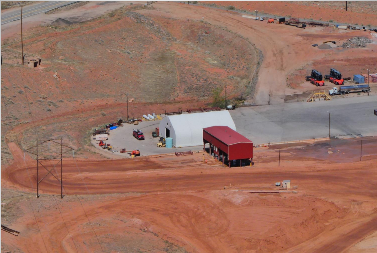
Lidding and Un-lidding Building (front) with Maintenance Building (behind)
