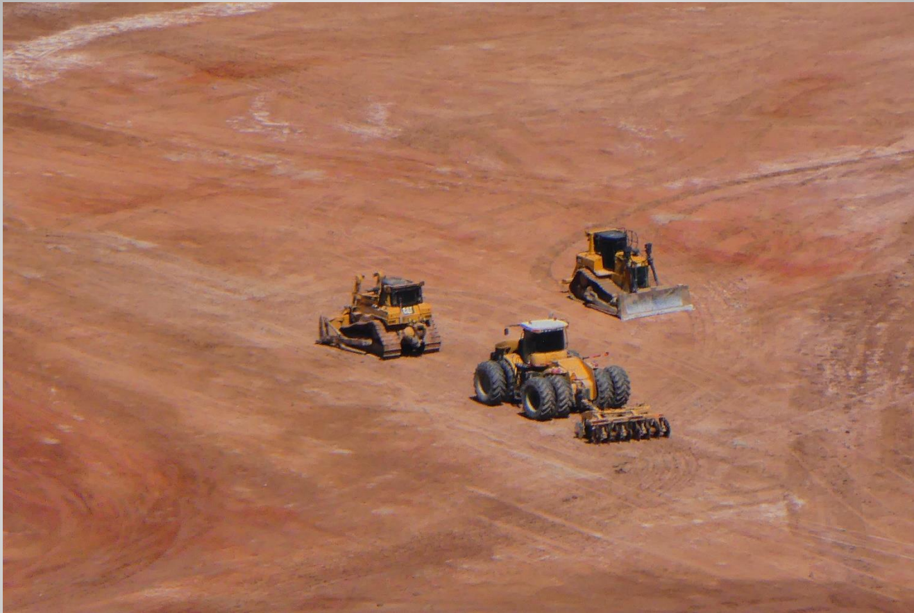
Close view of equipment used to prepare conditioning beds
