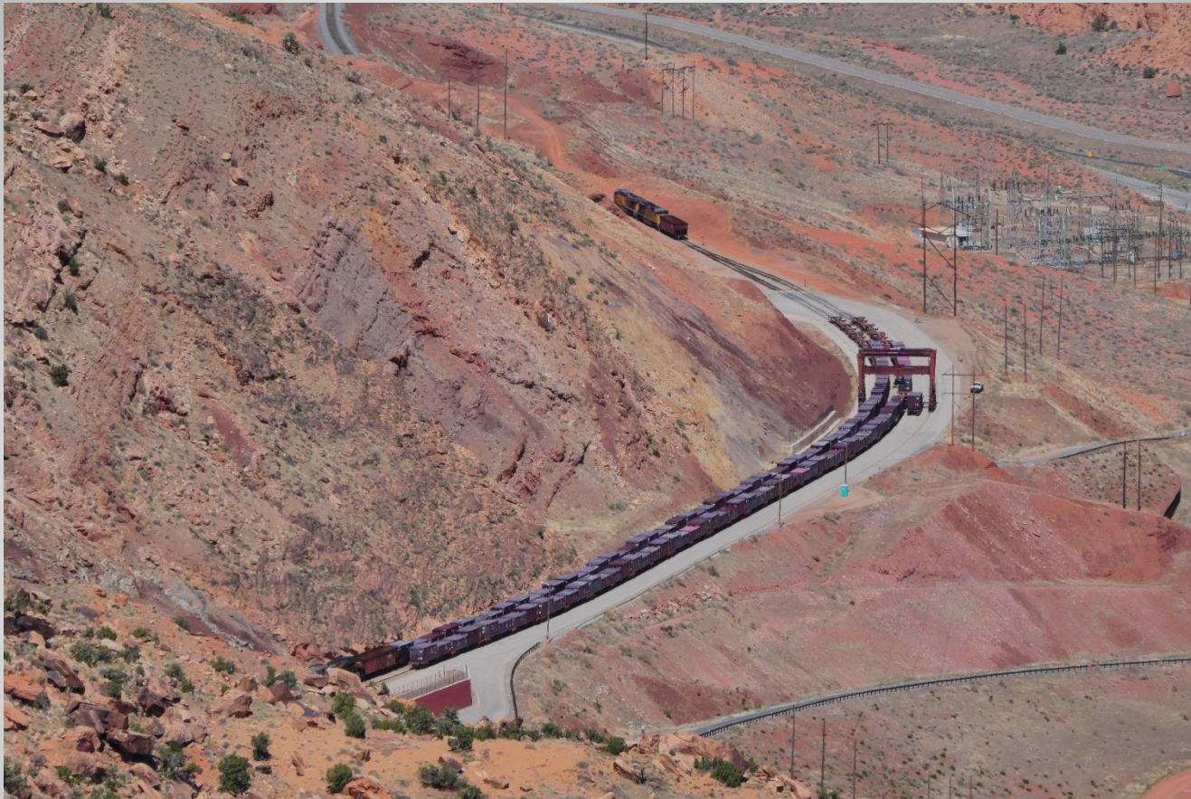
Rail Bench Loading Area Main Line (Left), Spur (Right)
